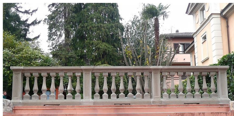
Balastra in cemento
